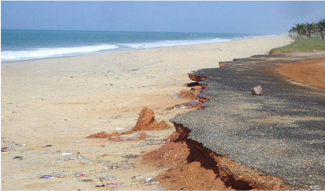
Figure 8: Coastal road infrastructure damage by sea erosion at Ada
